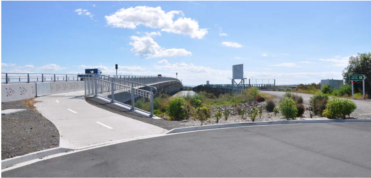
Photo 11: Pedestrian and cycle access over the new Kopu Bridge (left), and access to the old Kopu Bridge (currently closed) (right).
