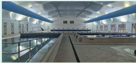
Opened in June 2024, the structural fabric building is a double-skinned PVC, fully insulated, over a steel structure. The building fabric has a service life of 15-30 years and a warranty of 15 years. The financial modelling has scheduled replacement every 20 years with additional cleaning every 12 months to keep the fabric free of mould and mildew.
